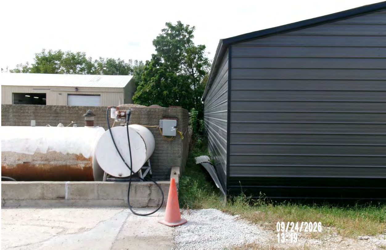
From adjacent property looking west along south property line.
