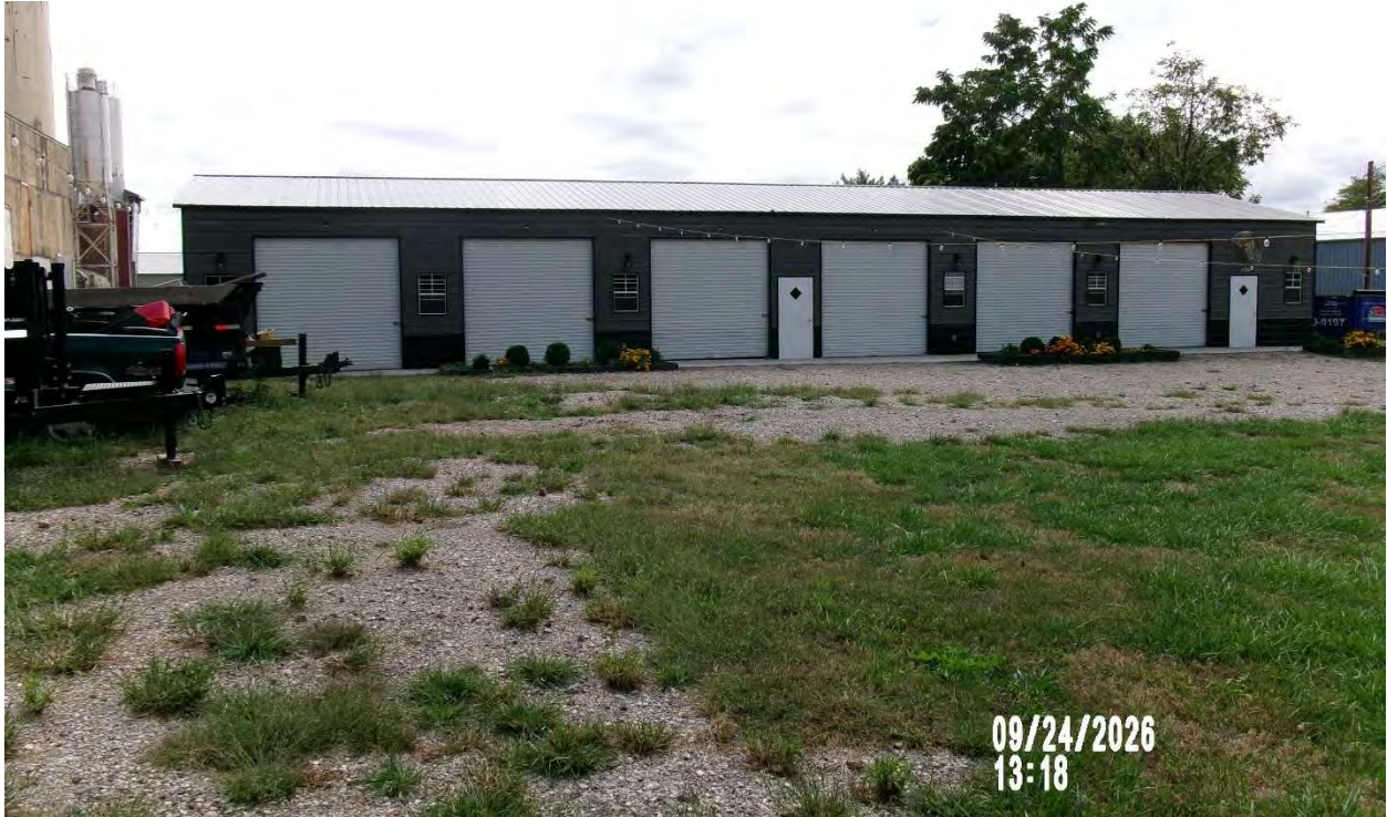
From the subject property looking south toward building.
