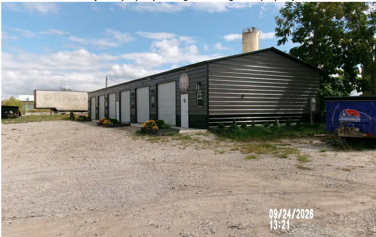
From subject property looking southeast toward building.
