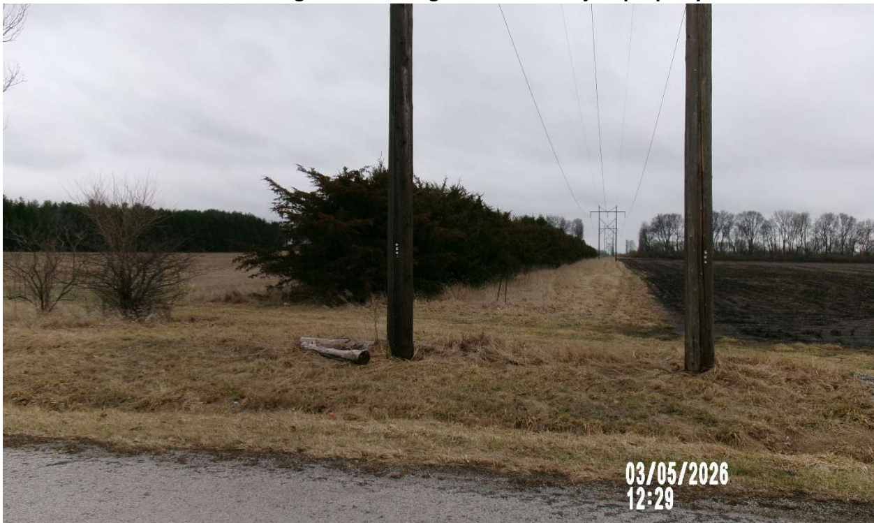
From Washington St. looking south along west property line
