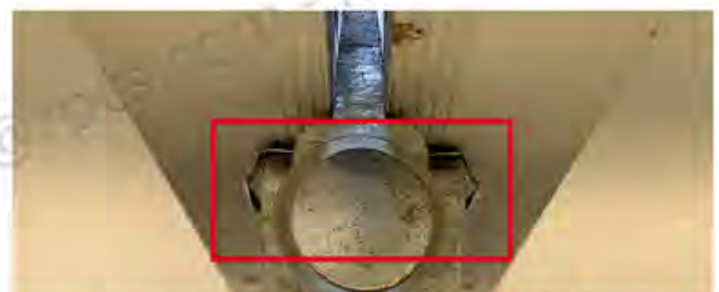
Figure 7-13: Grounding Clip Present on Module Clamp
