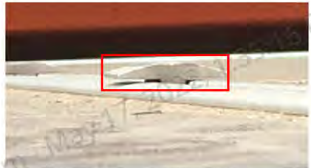
Figure 7-11: Clamp Ear Not Flush To Frame
