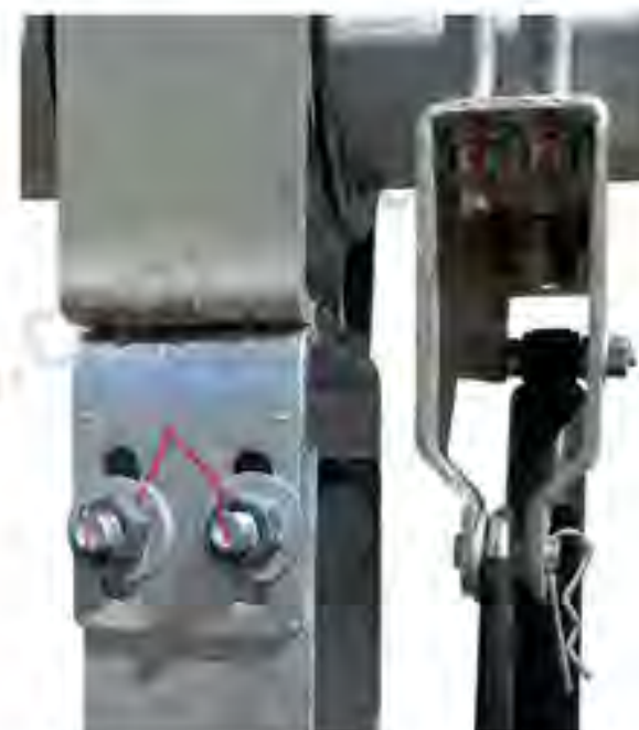
Figure 5-2: Proper Marking of Torqued Hardware
