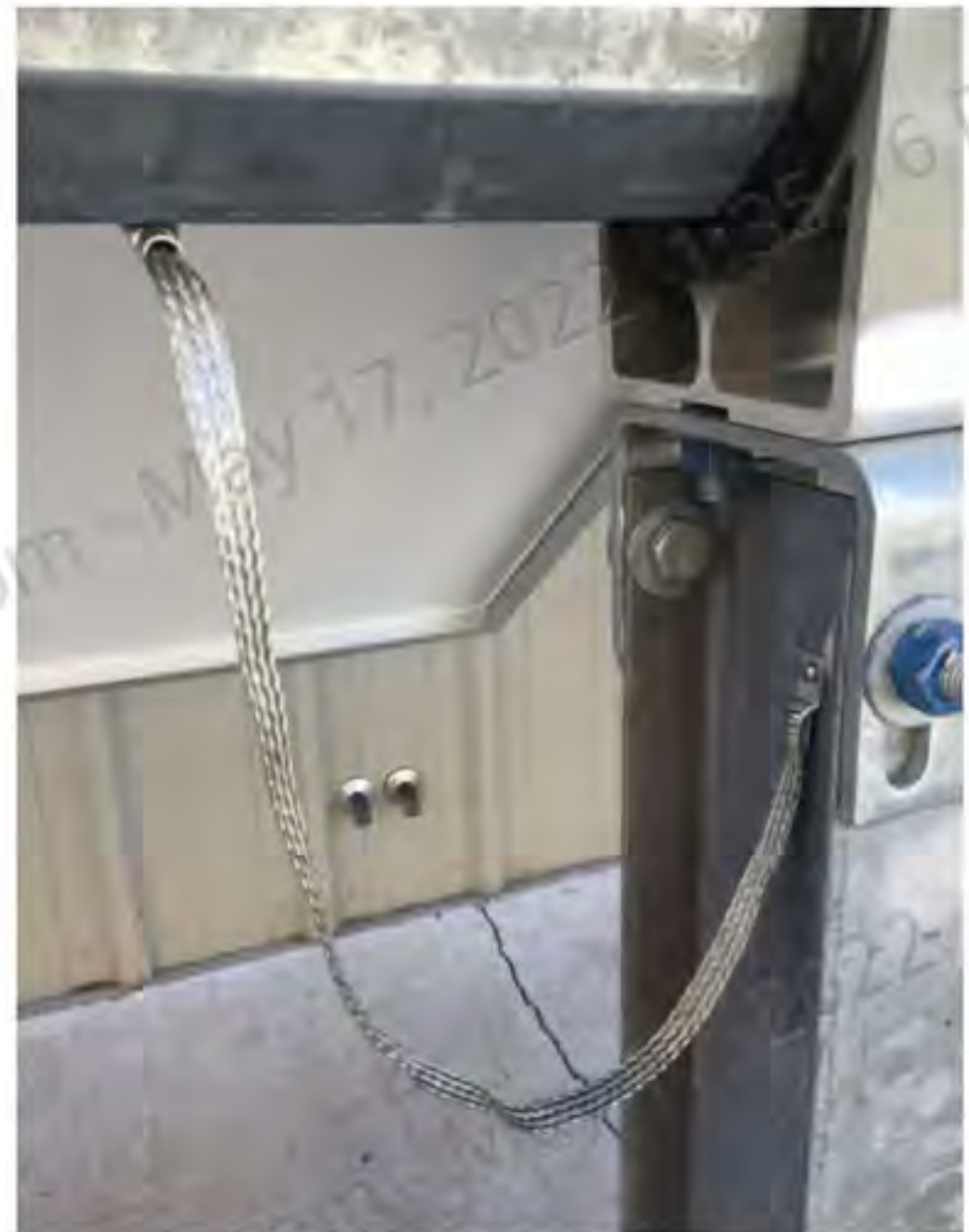
Figure 11-7: Installed Alternate Ground Cable
