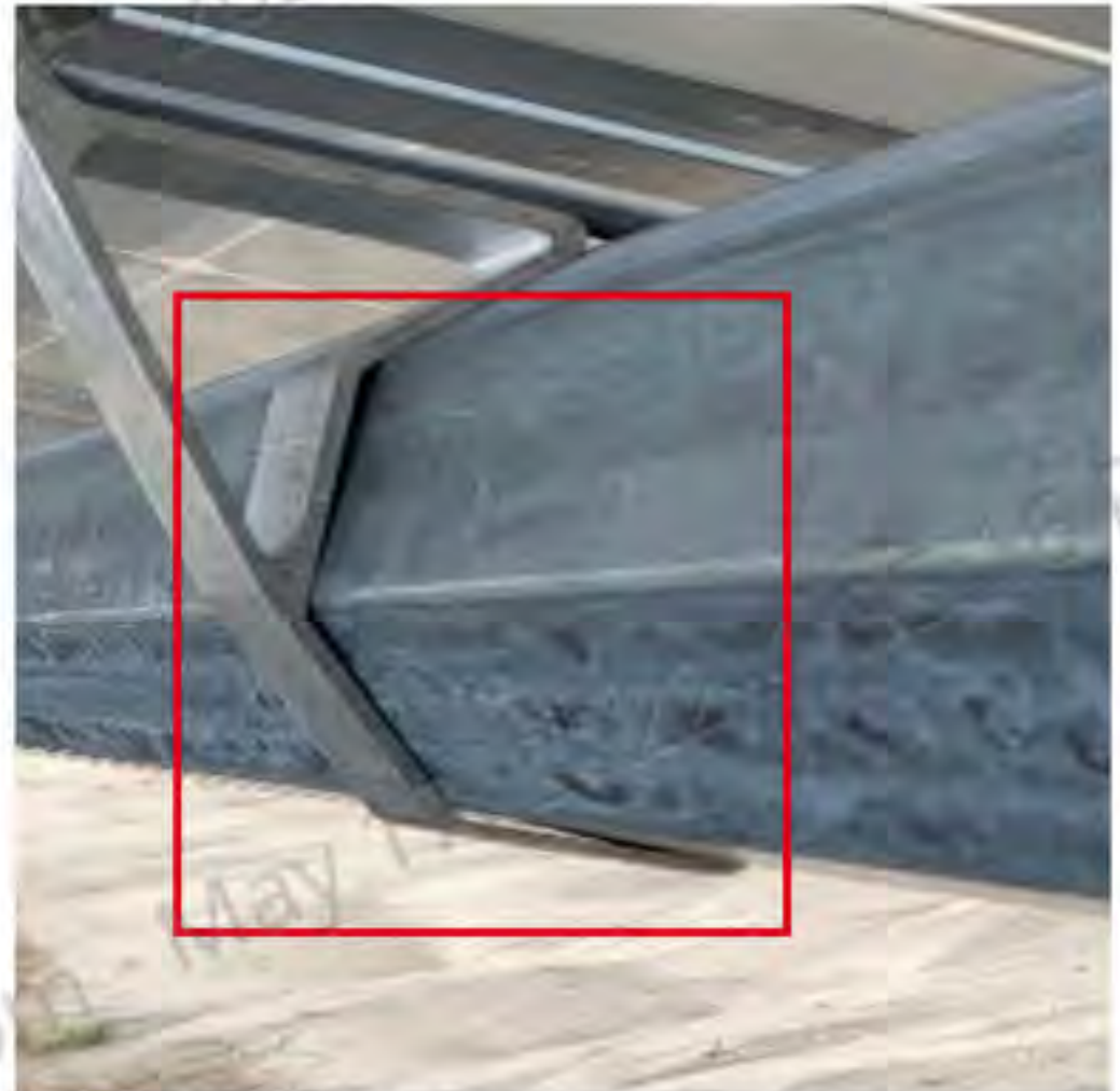
Figure 9-7: Module Clamp Positioned Incorrectly
