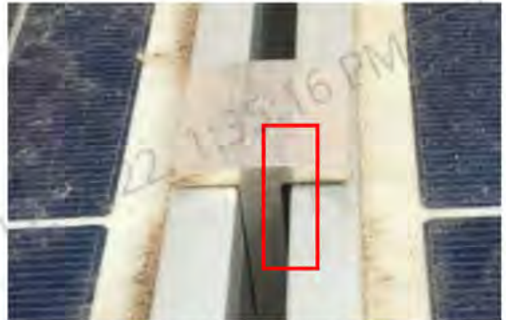
Figure 7-10: Clamp Ear Not Vertical; Tilt Suspected
