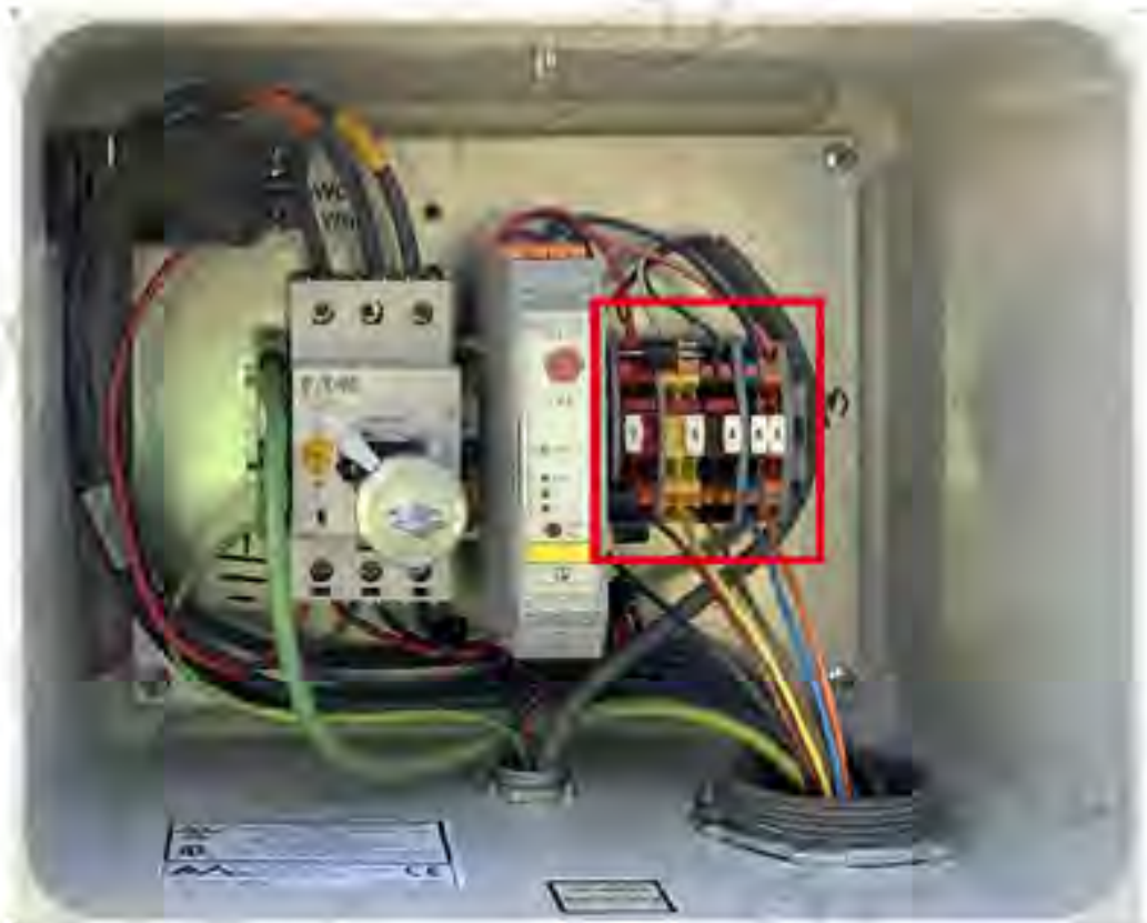
Figure 10-7: Example Motor Electronics Enclosure Interior (US)
