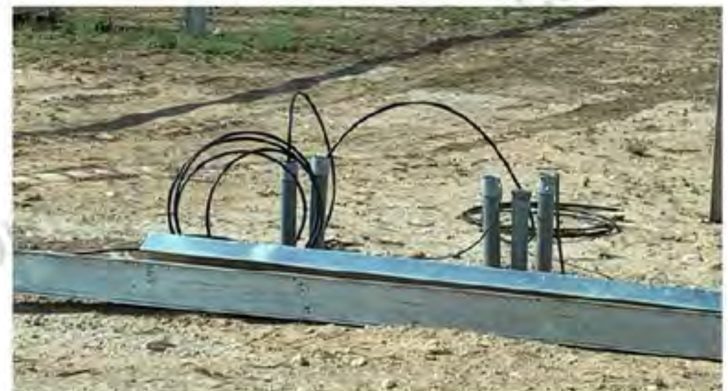
Figure 10-5: Bell Caps Protecting Control Wire From Abrasion
