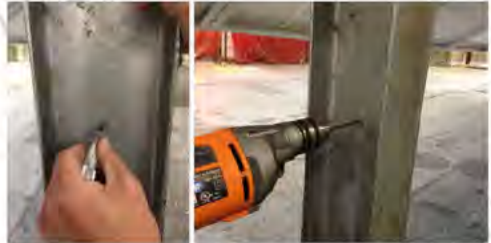
Figure 11-8: Grounding Lug Mounting Position (L) and Drilling (R)
