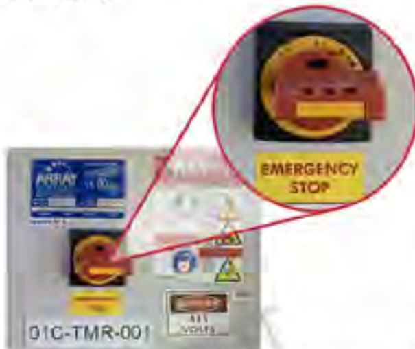
Figure 2-1: Emergency Stop Disconnect Switch
