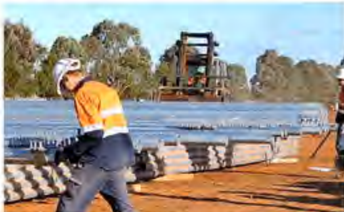
Figure 5-13: Torque Tube Pre-Assembly
