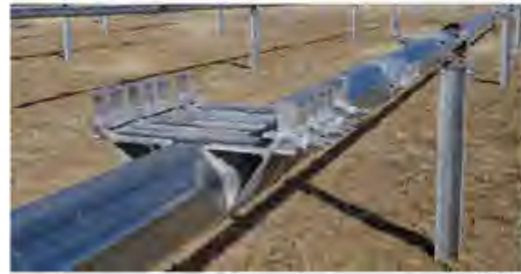
Figure 5-14: Torque Tube Placement on Support Column
