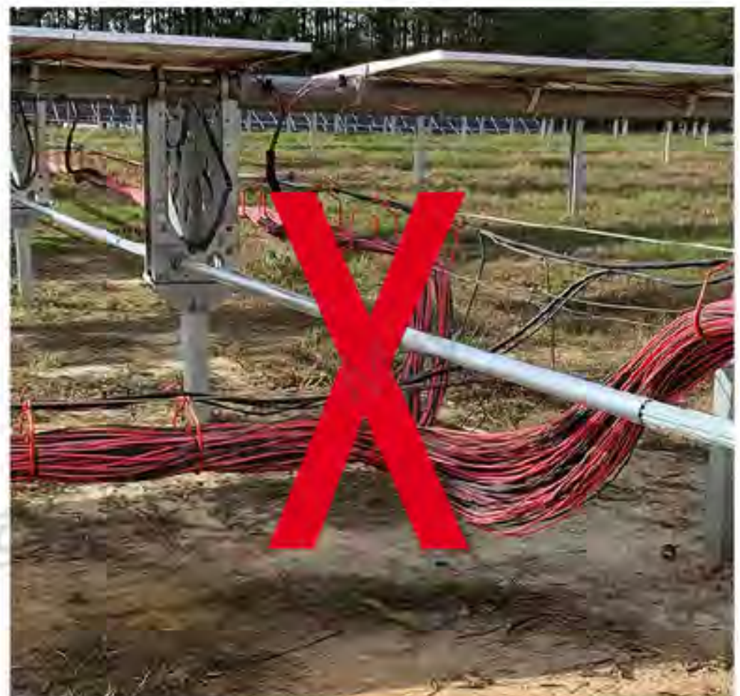
Figure 10-2: Wire Routed Hazardously Under Drivelines
