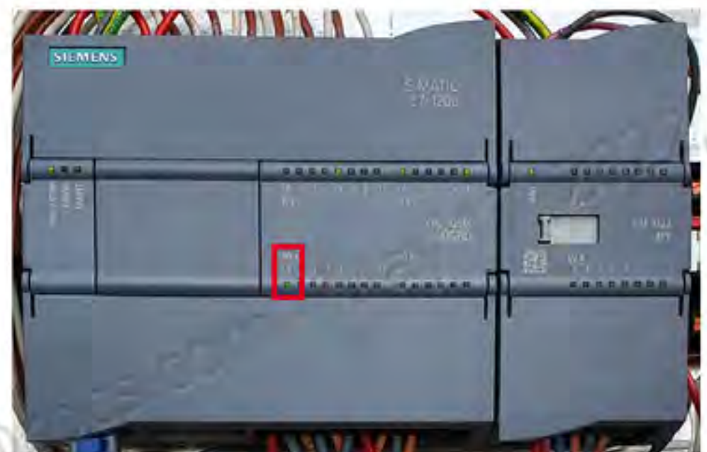
Figure 12-3: GPS Connection Indicator Light on PLC
