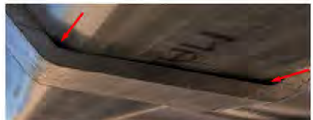
Figure 7-12: Clamp Body Not Parallel to Bottom of Torque Tube
