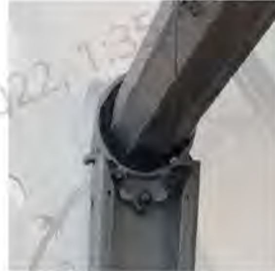
Figure 5-20: Center Structure Bearing Housing Aligned to Upright
