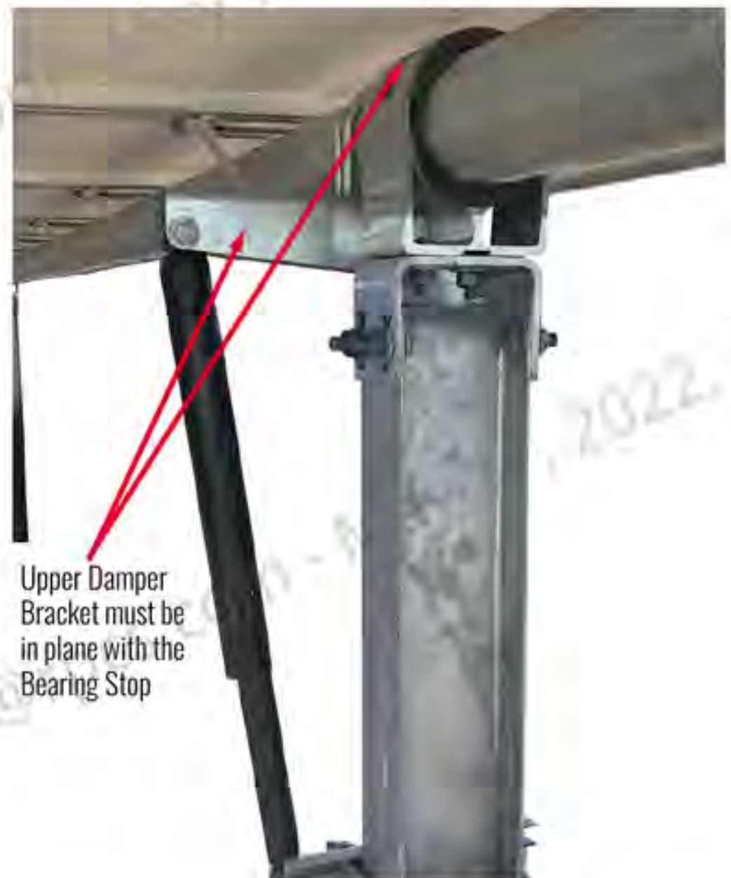
Figure 5-33: Damper in Plane with Bearing Stop
