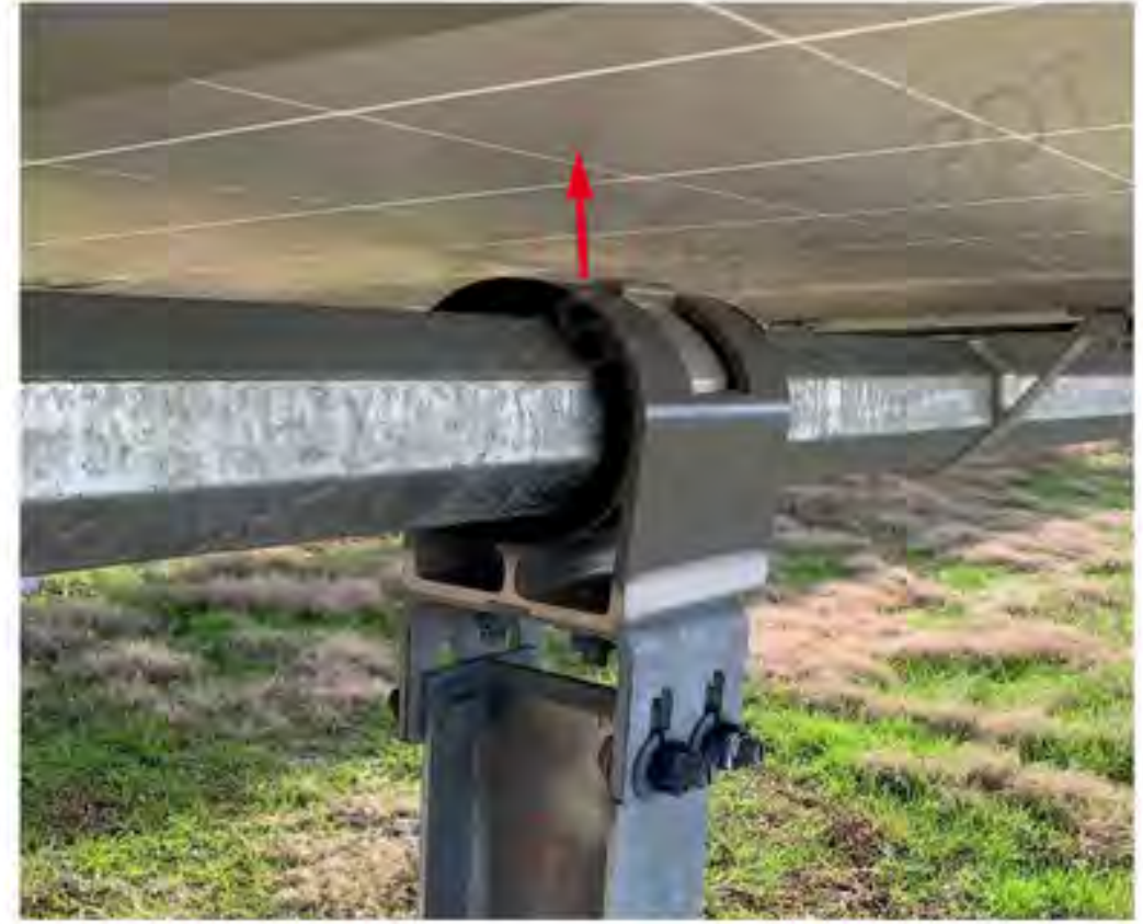
Figure 9-3: Bearing Housing Center Stop Seated Correctly
