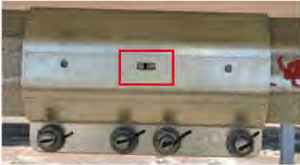
Figure 5-26: Coupler With Alignment Window
