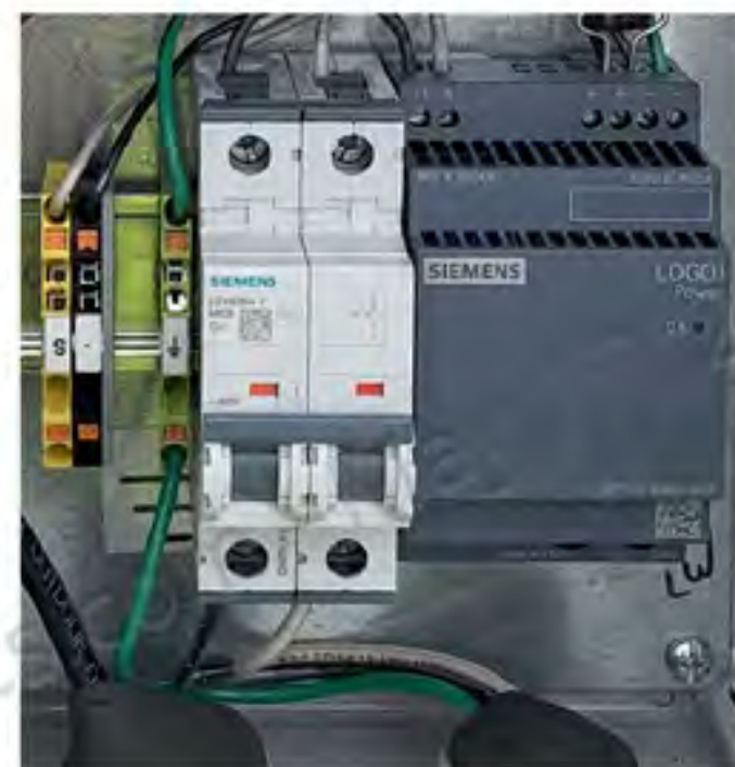
Figure 10-12: Ground (GRN) & Power Wires (B/W)
