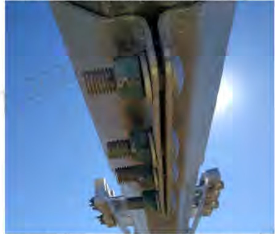
Figure 5-29: A Gap in the Flanges May Exist; Bolts Must be Seated
