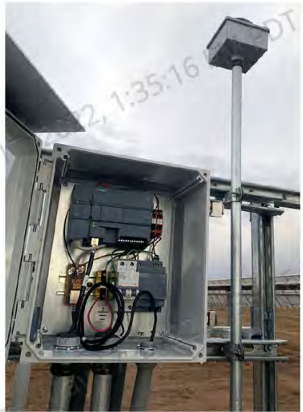
Figure 12-2: Site Data Controller & GPS Unit
