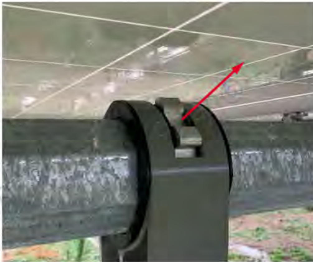
Figure 9-2: Bearing Housing Center Stop Seated Incorrectly
