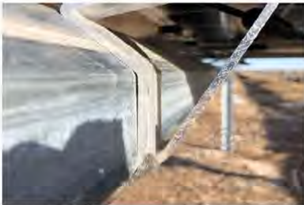
Figure 7-6: Slight Gaps Between Certain Clamp Arms Are Possible
