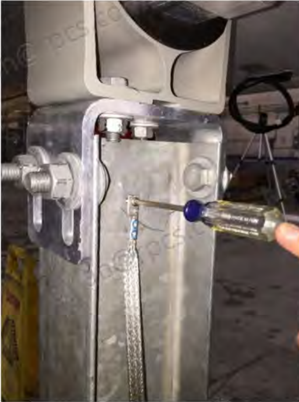
Figure 11-6: Ground Cable Installation
