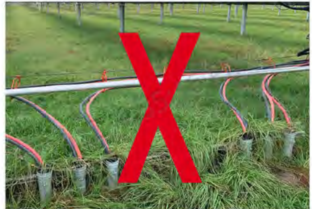
Figure 10-4: Hazardous Stub-out Placement Near Drivelines
