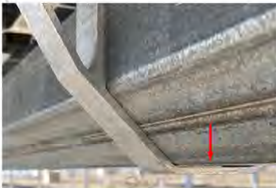
Figure 7-7: Slight Gaps Between Certain Clamp Arms Are Possible
