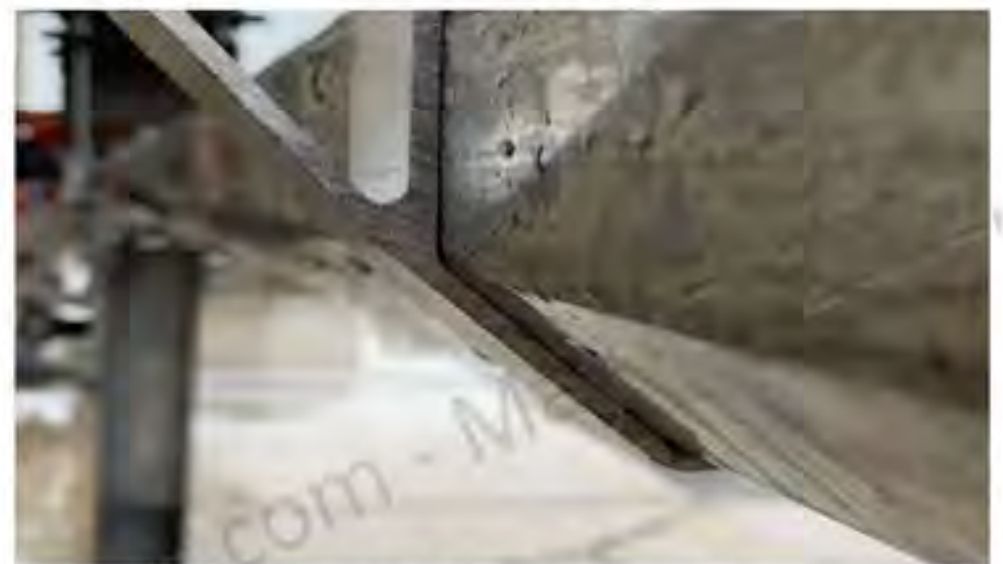
Figure 9-8: Module Clamp Positioned Correctly
