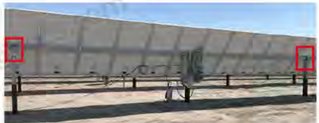
Figure 5-11: Bearing Housings With Set Screws Location
