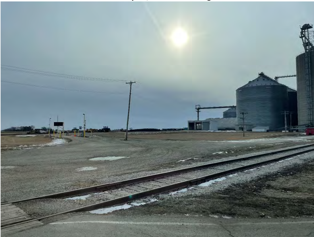
From the NE corner of the Subject Property looking SW
