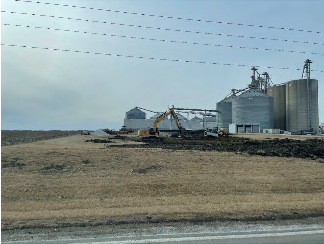
From Co Hwy 23/CR 950E looking west
