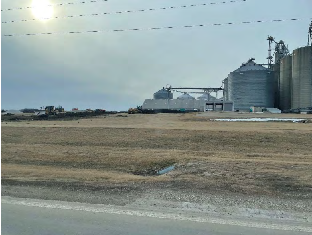
From Co Hwy 23/CR 950E looking west
