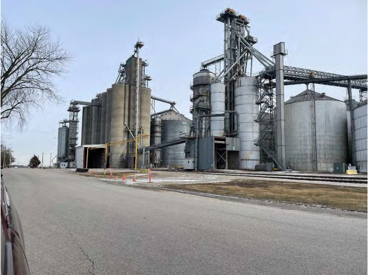
From Second St. looking SE toward Subject Property
