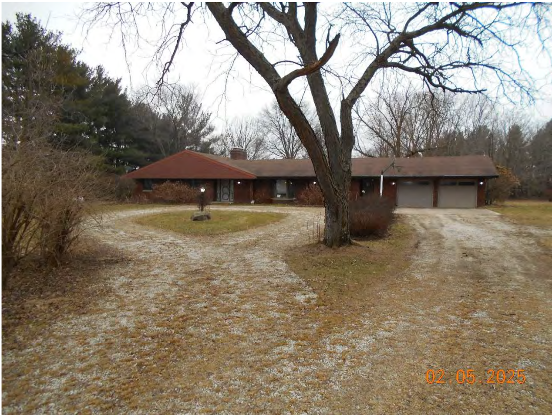
Looking south on the subject property toward the residence
