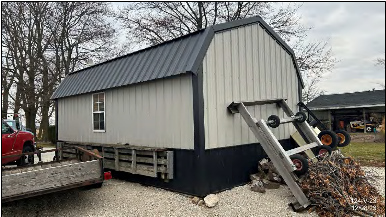
From edge of cultivation line facing NE to shed – distance is 16 feet
