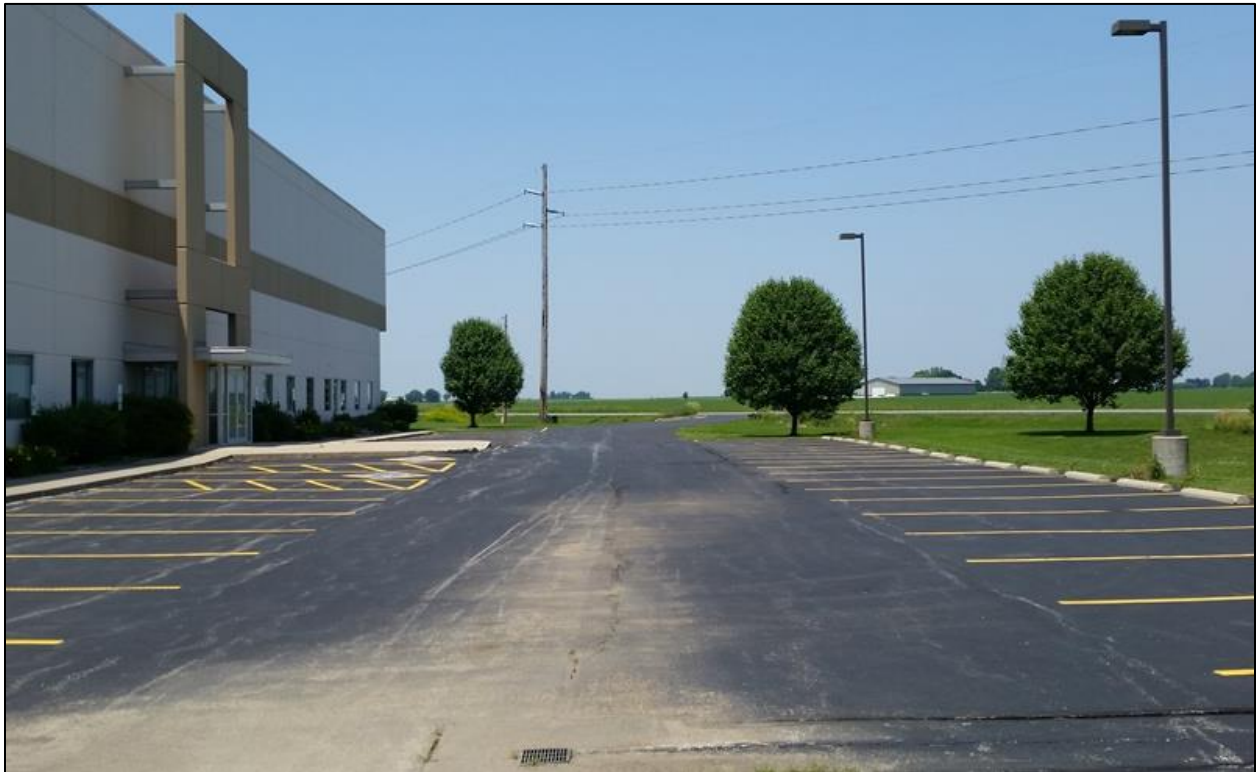
Existing parking lot facing northwest toward existing property access (2015)
