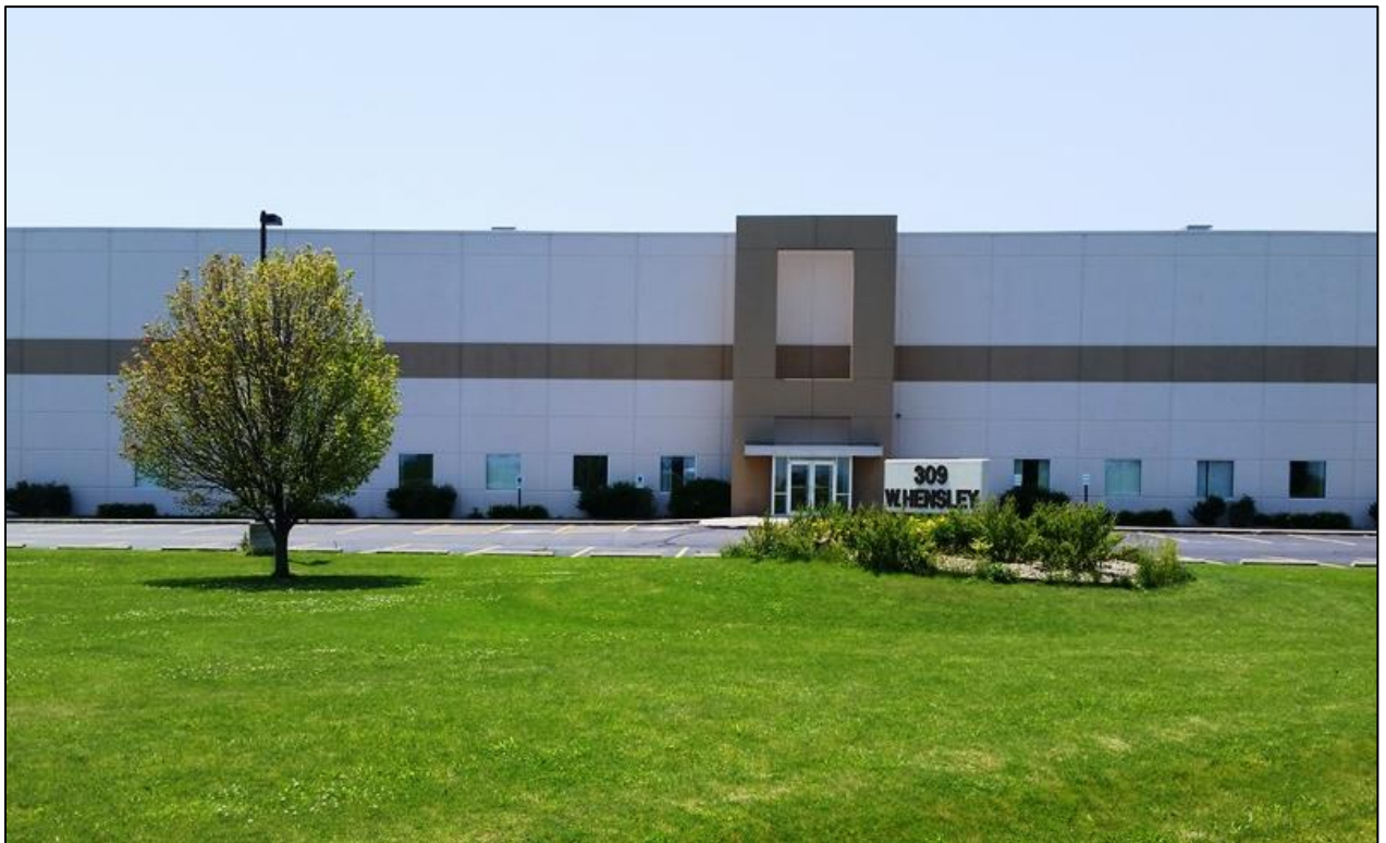
From Hensley Road facing existing Rush Truck Center (2015)
