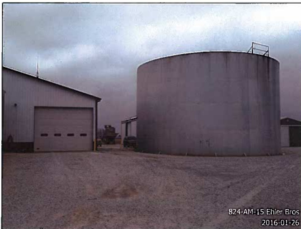
Existing Ehler Bros facility liquid fertilizer storage tank
