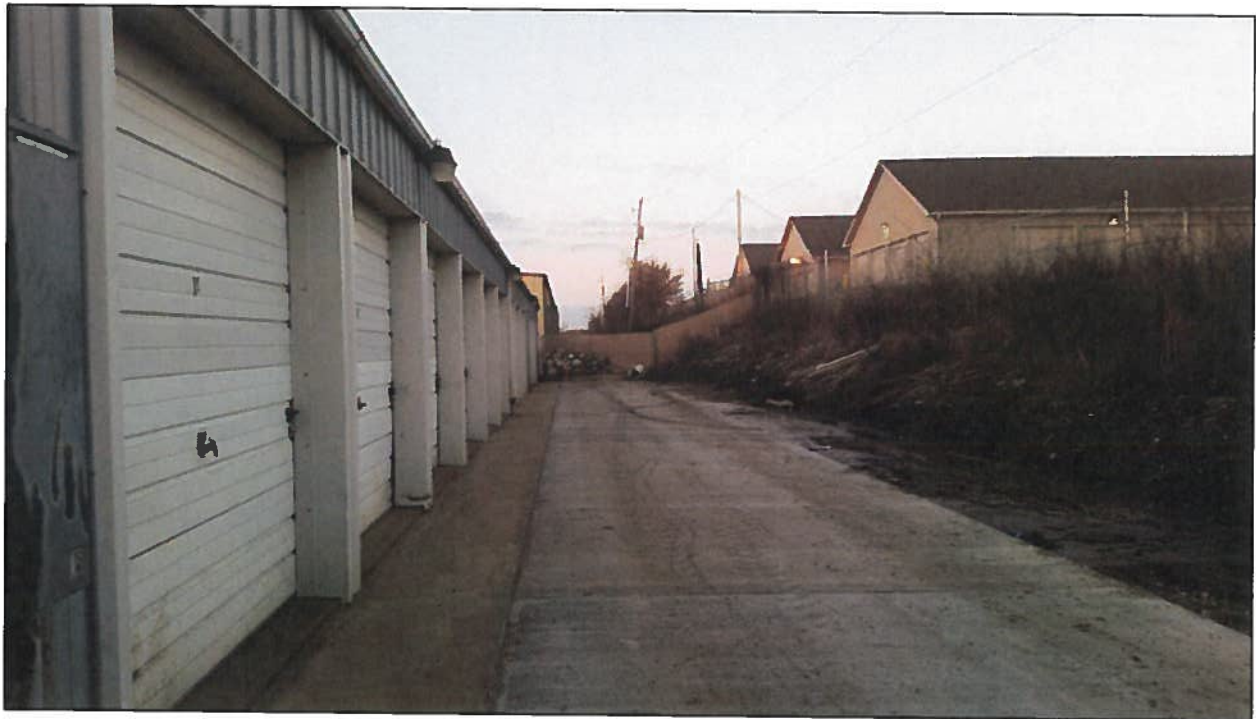
East side of storage area facing north from driveway
