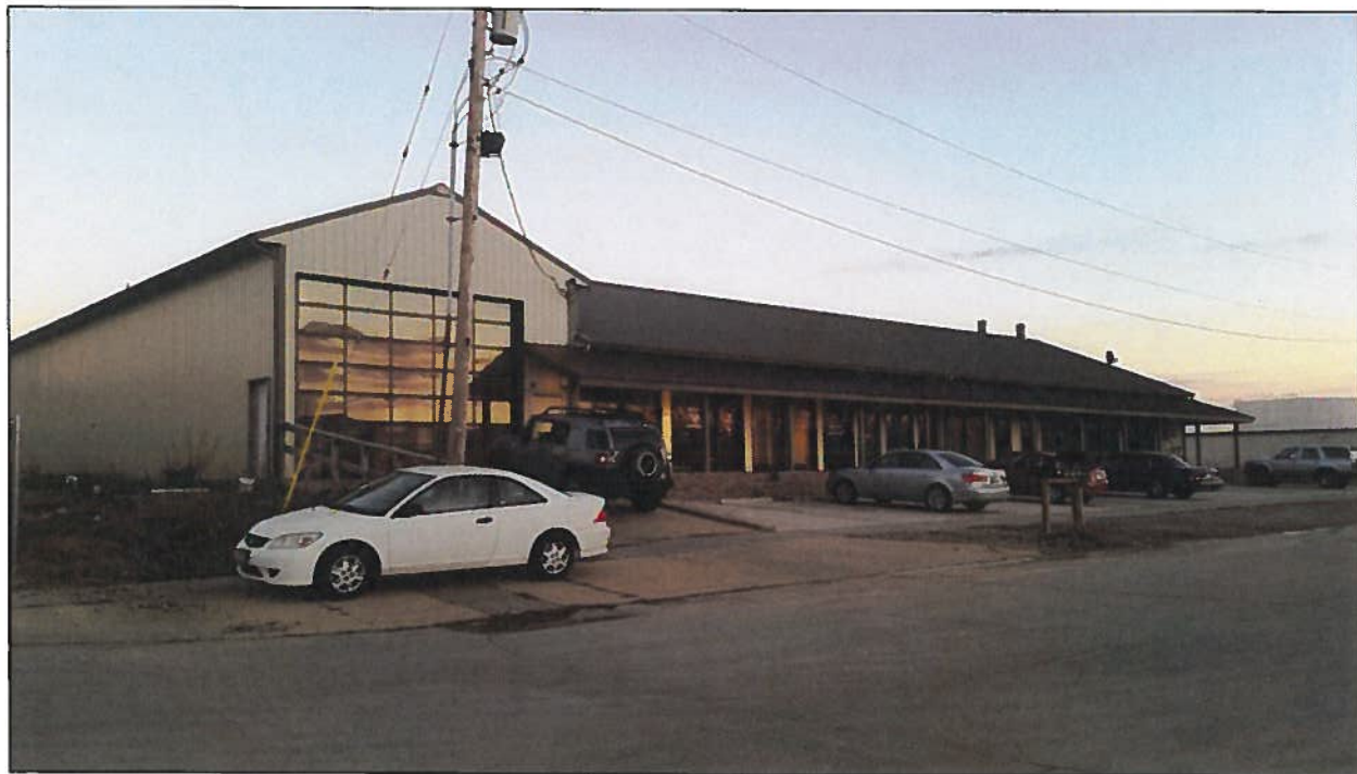
Offices on west end of property, from Tiffany Ct facing southeast
