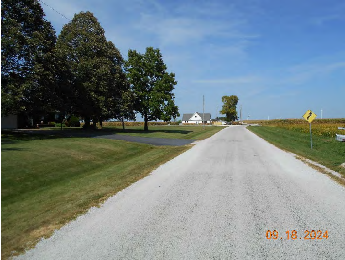
Facing North along 2600E
