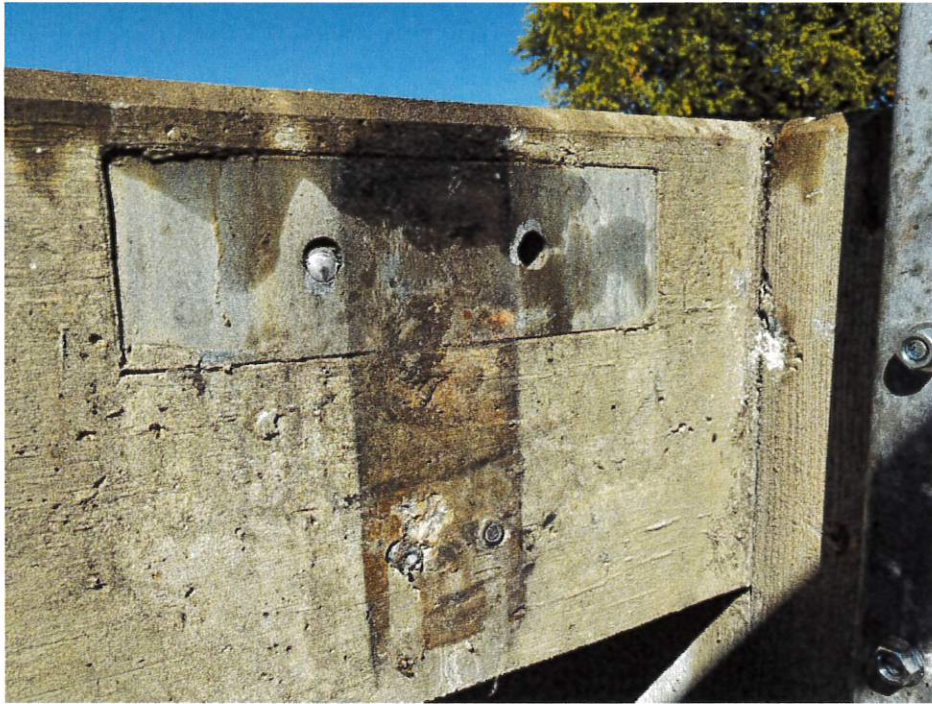
Post One – Post obliterated and Bolts missing or sheared
